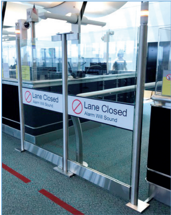
Alarmed doors install at Newark Intl. Airport Terminal B.
