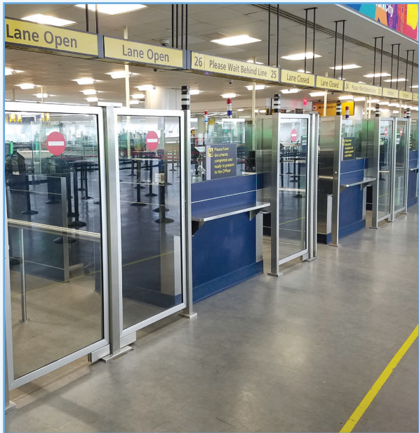
Alarmed doors install at JFK Intl. Airport T1.
