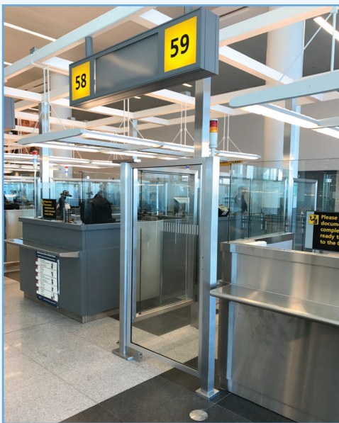
Alarmed doors install: JFK Intl. Airport T4.
